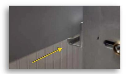
4. BE SURE TO LEAVE SPACE BETWEEN THE BOTTOM OF THE DOOR GUIDE RAIL AND BRACKET.
