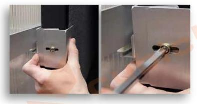
5. ONCE IN PLACE, SECURE THE BRACKET BY SQUEEZING AND TIGHTENING THE SCREW WITH A PHILLIPS SCREWDRIVER.
